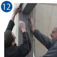
**12** Tape string (tape string to face of frame in opposite corners running diagonally) to check alignment of frame. Keep in mind you may need to move one string from inside to the outside to make sure of correct alignment.
