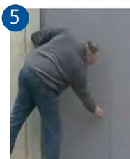
**5** Check for appropriate gaps between door and frame. Refer to NFPA 80 for correct clearances. Shim if needed. See Steel Door Institute publication 122-07 for shimming instructions.
