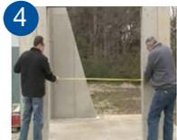
**Note:** The installer is responsible for shimming and aligning the frame. Gaps are normally sealed as part of the installation or caulking/painting process. Refer to architectural specifications for the appropriate sealant material to be used at fire or smoke control openings.
