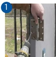
**1** Install hinges onto door using manufacturer's instructions. Use screws provided with hinges. DO NOT SUBSTITUTE.
