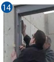
**14** Plumb and square the strike jamb, and shim if necessary. Shims used should be located immediately above the anchor points.
